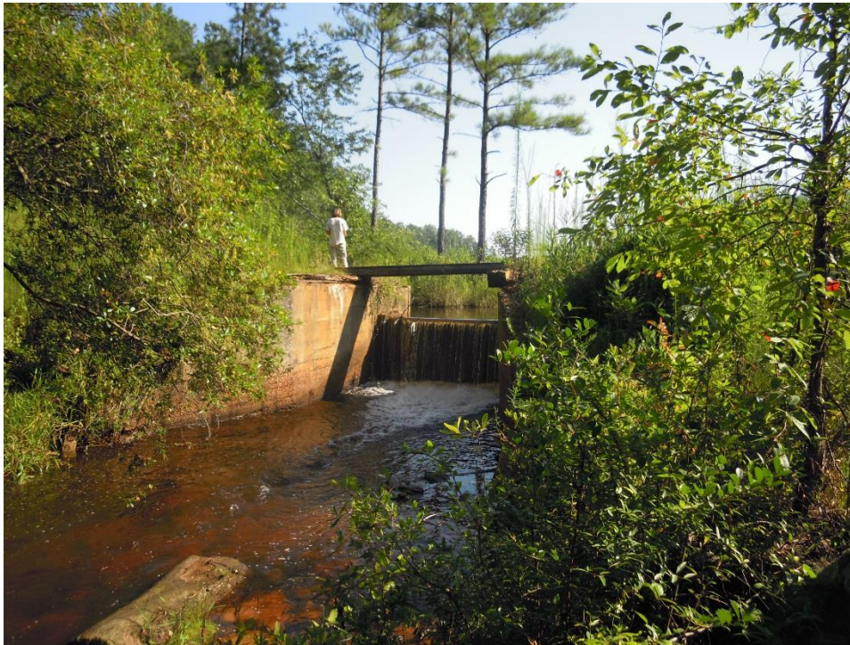
Figure 10. The spillway from the downstream side of the dam.
